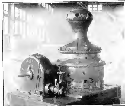
Pelton water wheel driven Hyde dock capstan specially designed for use on oil wharf at Richmond, California.
